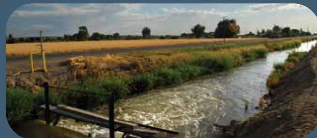
LINING AND COVERING CANALS PREVENTS EVAPORATION AND GROUND LOSS
